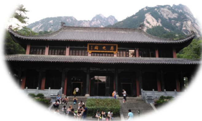
Figure 2-2 Huangshan CiGuang Pavilion
