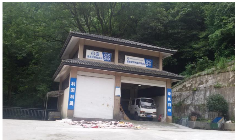
Picture 5-2 Wenquan Waste Transfer Station
