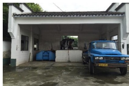
Figure 7-3. Waste transfer station
