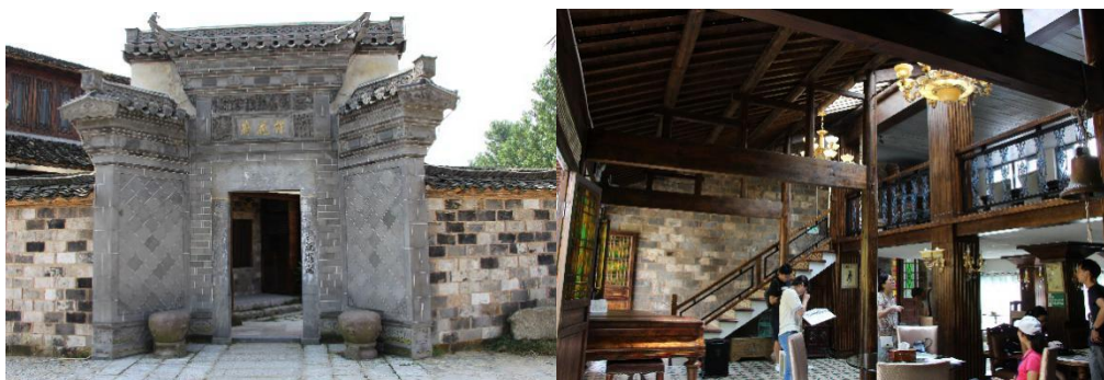
Figure 2-4 Entrance gate house and internal decoration of Tanhua Mansion
